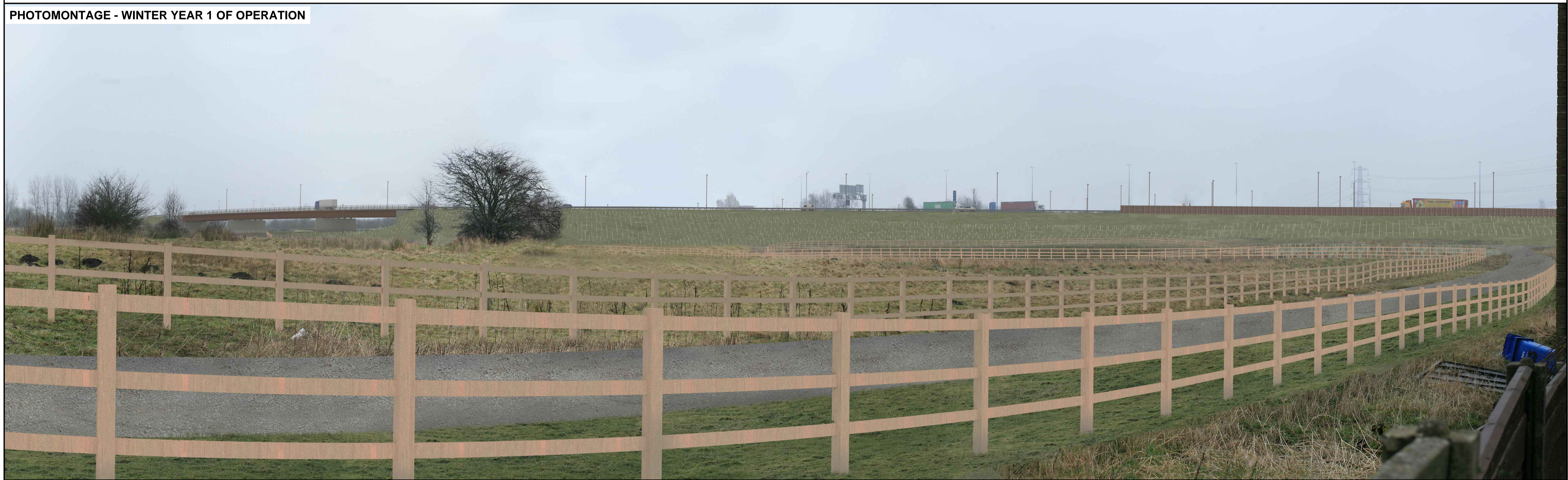
VIEWPOINT PM02: View looking east from Marston Close in Whitefield to the Simister Pike Fold Viaduct and new embankment.
